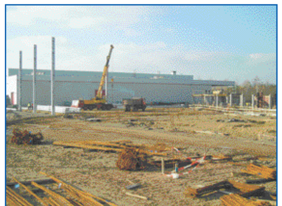
Construction site in Poland
