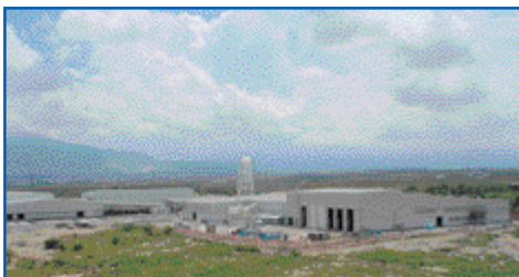
Camisa, new foundry in Saltillo, Mexico
