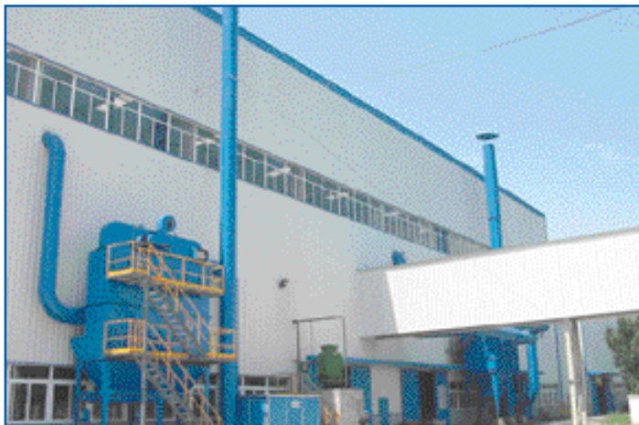
New facility, filter area sand plant and sand drying system
