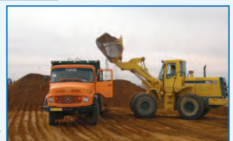
Excavation works in February 2007
