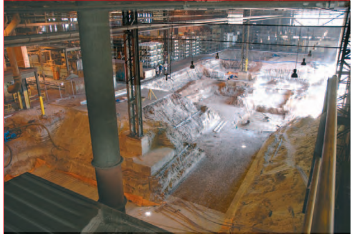
Preparation, civil works for moulding line
