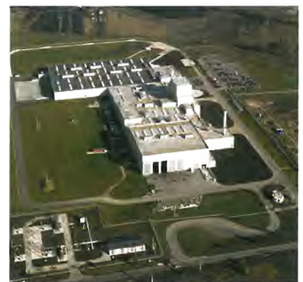
Foundry and machining facility of Wescast, Oroszlány, Hungary, as built in 2001. The production facility manufactures exhaust manifolds, turbocharger housings and integrated turbo-manifolds
