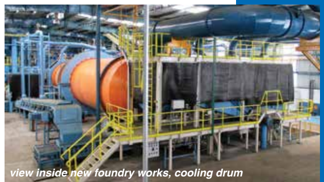
New foundations for state of the art foundry operations
