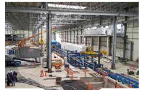
The dynamics of a greenfield casting facility in the making, with sand plant in construction on the outside and the casting line taking shape on the inside (melting, pouring).
