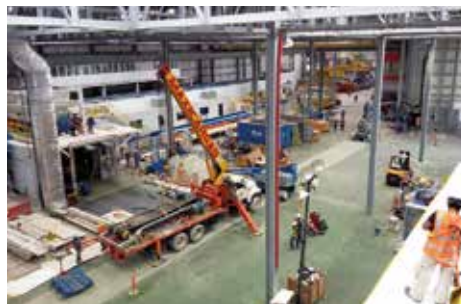
The dynamics of a greenfield casting facility in the making, with sand plant in construction on the outside and the casting line taking shape on the inside (melting, pouring).
