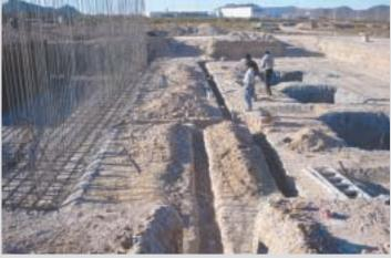
work in progress, excavation works for grounding system
