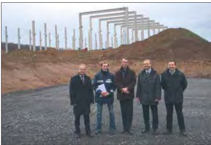
“Construction ongoing” From left to right: Mr. Rolf Behringer, Mr. Maurits Brandt (Gemco), Mr. Cees Noortman (Gemco), Mr. Christian Behringer, Mr. Dieter Karasek (Behringer)
