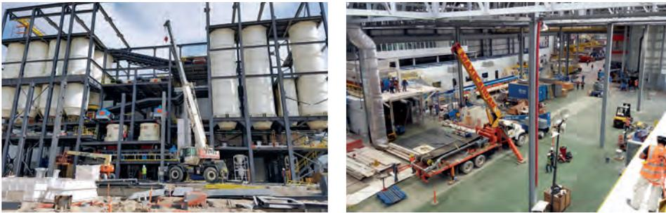
*The dynamics of a greenfield casting facility in the making, with sand plant in construction on the outside and the casting line taking shape on the inside (melting, pouring).*
